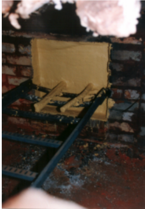
Figure 3: Installation prior to test as seen from the inside
