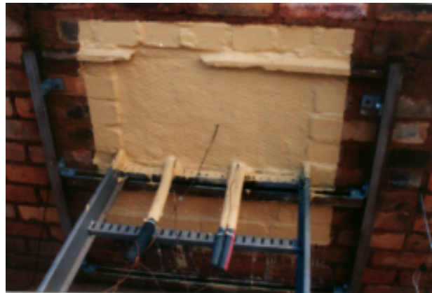
Figure 2: Installation prior to test as seen from outside
