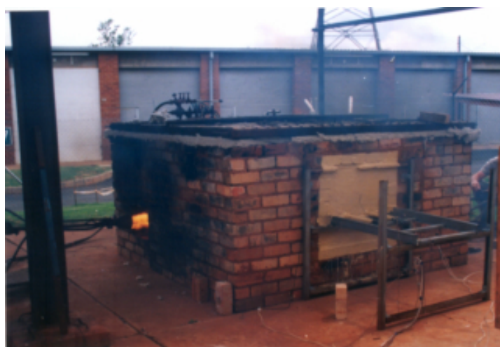
Figure 5: Diesel burner on lefthand side in operation
